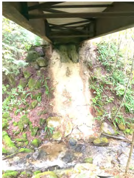
Left Bank Abutment when facing downstream
