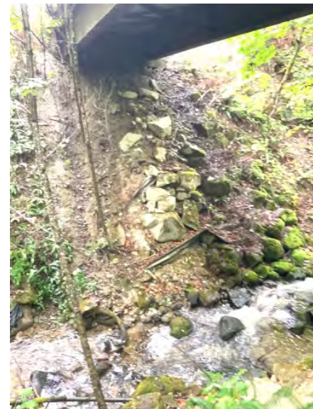
Right Bank Abutment when facing downstream
